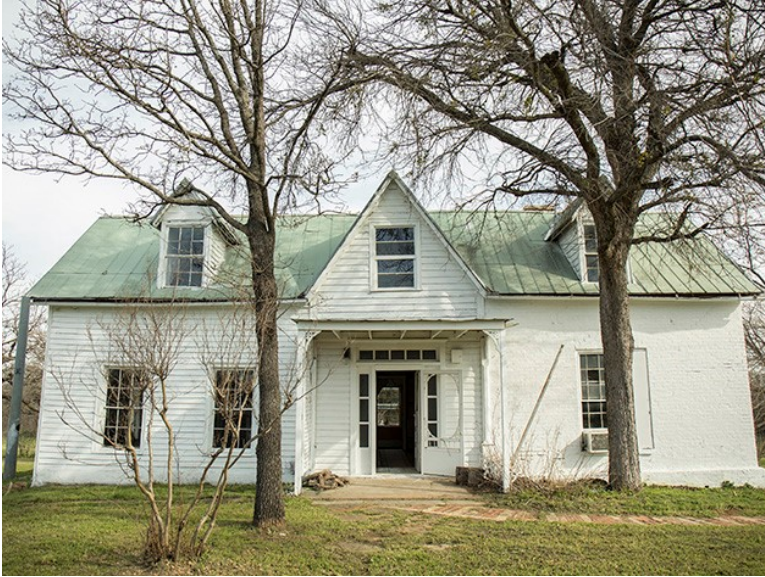
Figure 2-1. The Ralph S. and Julia B. Man House is a well-crafted, mid-nineteenth-century residence that was listed in the National Register of Historic Places in 2003. The property is a well-preserved example of a house that was popular in much of Tarrant County at that time; however, it is only one of few extant examples from that era to survive the county’s subsequent growth and development. The original log cabin remains beneath the cladding to the left of the main entry. Source: City of Mansfield.
