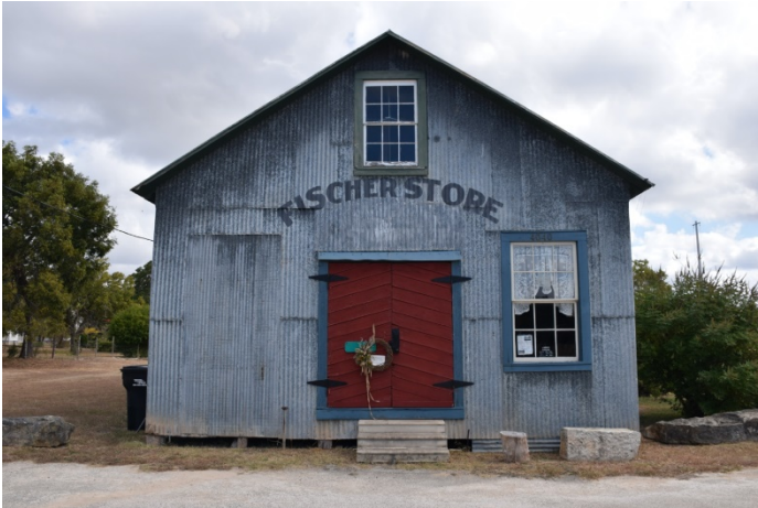
Figure 4-3. The Fischer Historic District in rural Comal County includes a dispersed rural settlement clustered around the Fischer General Store and the old Fischer School House. Prepared under a CLG-funded grant, it includes a grouping of historic buildings in a setting that is experiencing rapid growth and development. The Comal County CLG program sought to pursue National Register designation because of the perceived threat of change and demolition due to suburban developments and an expanded road network. The designation has instilled renewed pride among the residents of Fischer who have celebrated the historic designation and are revitalizing their places of work and residences. It is the only historic district in rural Comal County. Source: THC.
